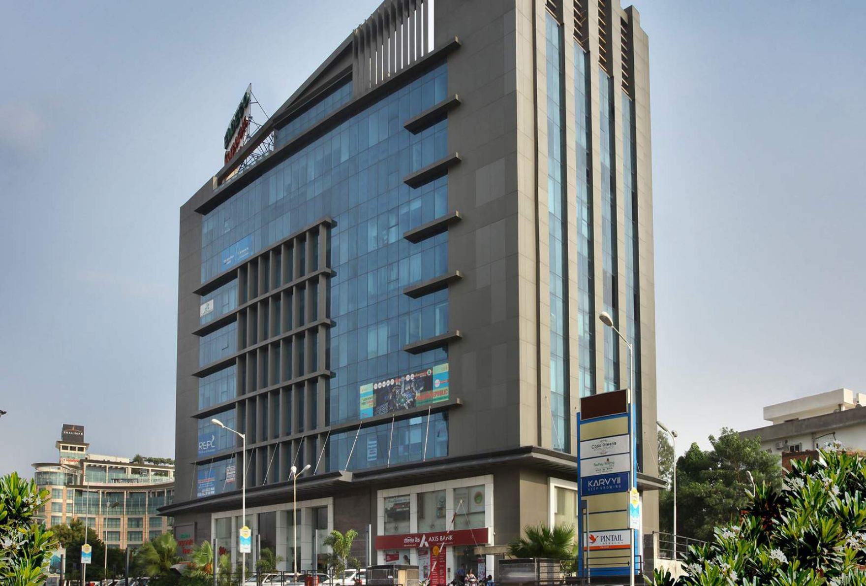
Eldeco Corporate Tower , Vibhuti Khand, Gomti Nagar, Lucknow
